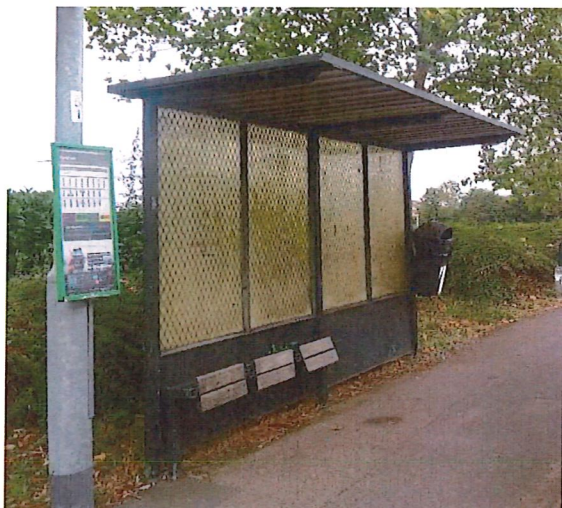
Old style shelter before renovation.
