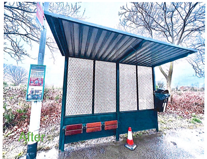
Old style shelter after renovation.
